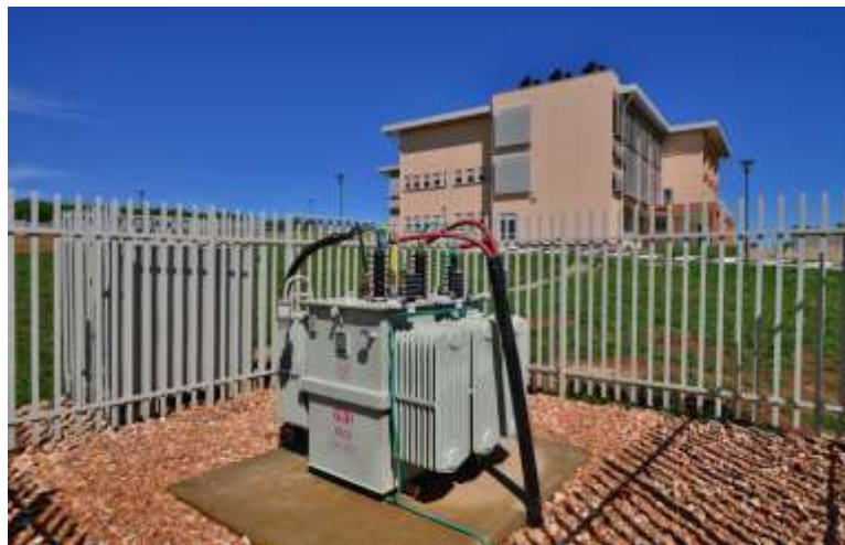
Supply, delivery and installation of Transformer
