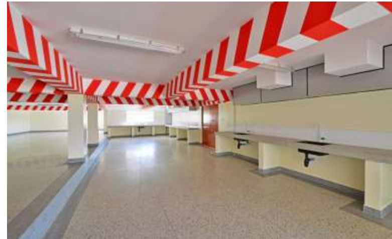
Basement of the Laboratory block
