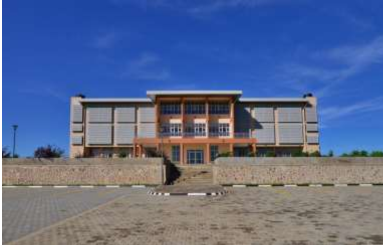
Main building front view
