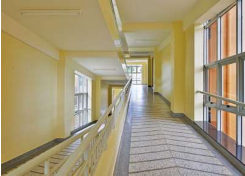
Ramp for people with disabilities
