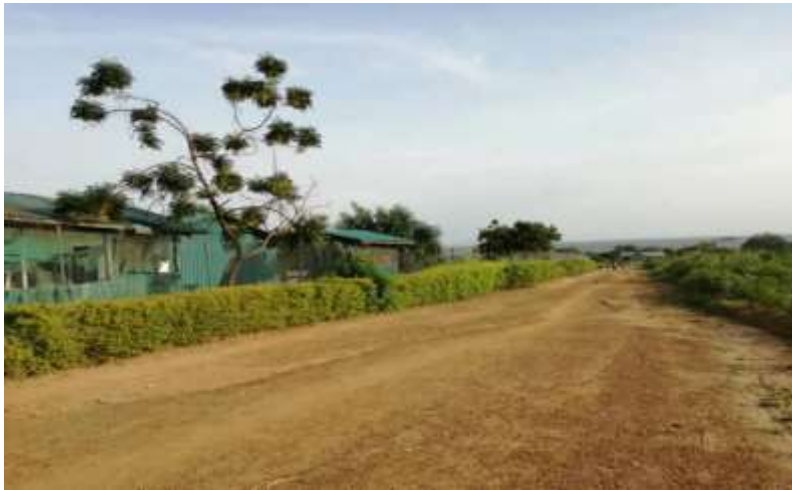
Access road created to the camp
